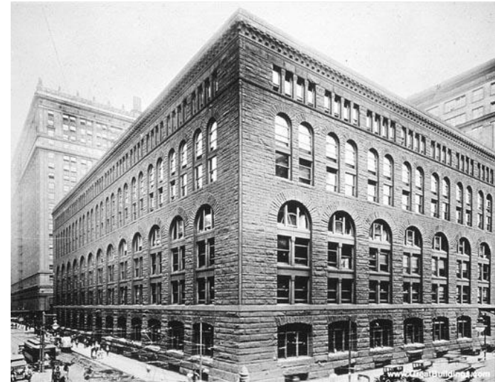
Marshall Field Warehouse Building . Henry Richardson, 1885-1887.
